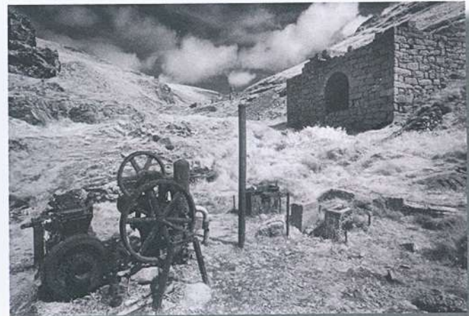
Mine Workings , Cape Cornwall - Nick Bodle Circle 10
